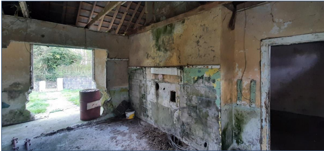
Plate 4-7 Interior of derelict dwelling - Exposed wooden beams and open loft space.
